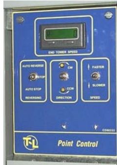
Point Control Panel
